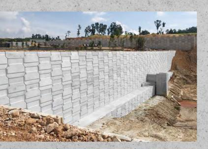
AnchorSOL Wall is externally clad with an aesthetically pleasing precast concrete finishing. Various selection of texture finishing choices is possible for consideration according to client's requirement.
